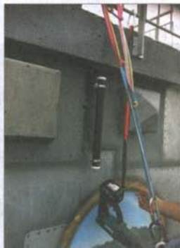
HB9BBD/B antennas: From left to right 6 dipoles for the 1296.050 MHz beacon, a slotted WG in the black tube for the 3cm beacon in 10368.063 MHz, and 6 dipoles for the 2320.050 MHz beacon.
